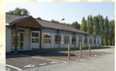
Restaurant scolaire Robineau
