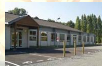
Restaurant scolaire Robineau
