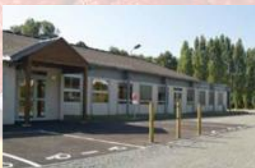
Restaurant scolaire Robineau
